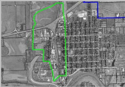
Aerial View of Site
