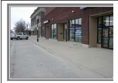
A curb cut that is no longer needed
